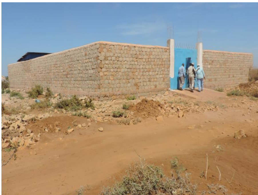
Completed stone rubble fencing © IOM 2018
