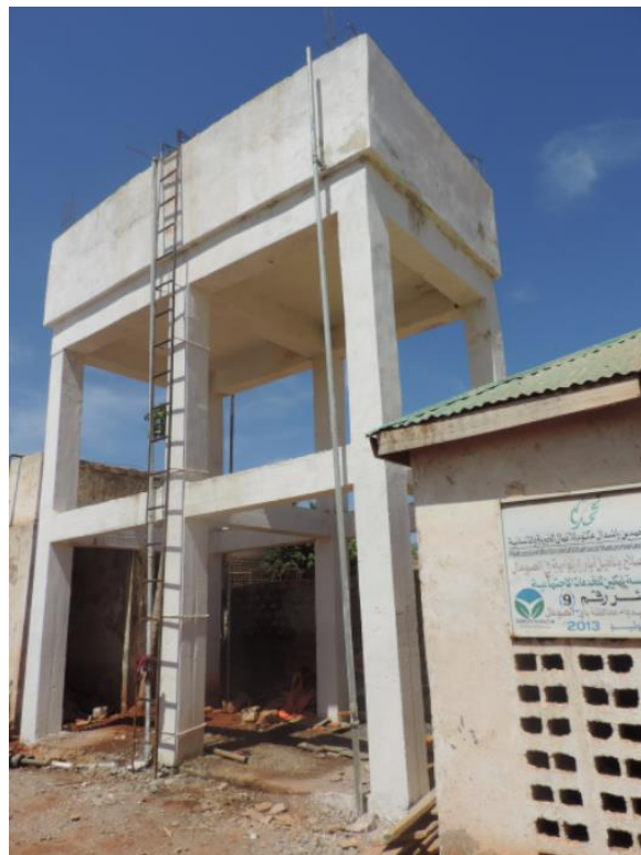
Completed elevated water tank © IOM 2018
