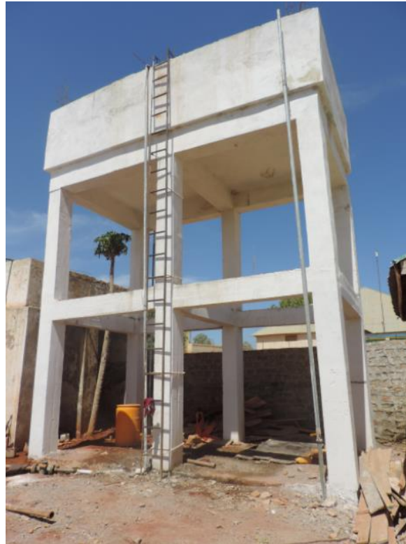
Completed elevated water tank © IOM 2018
